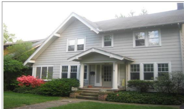
2822 Berkshire Road - View from Street
